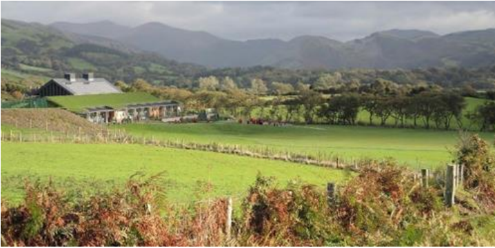
Image credit: Geraint Robert B3 Architects
