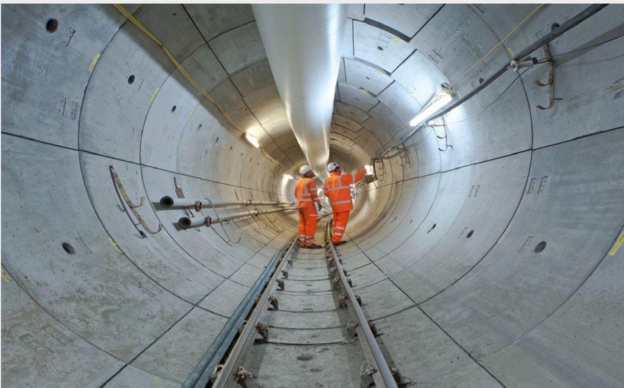
London Power Tunnels phase 1
